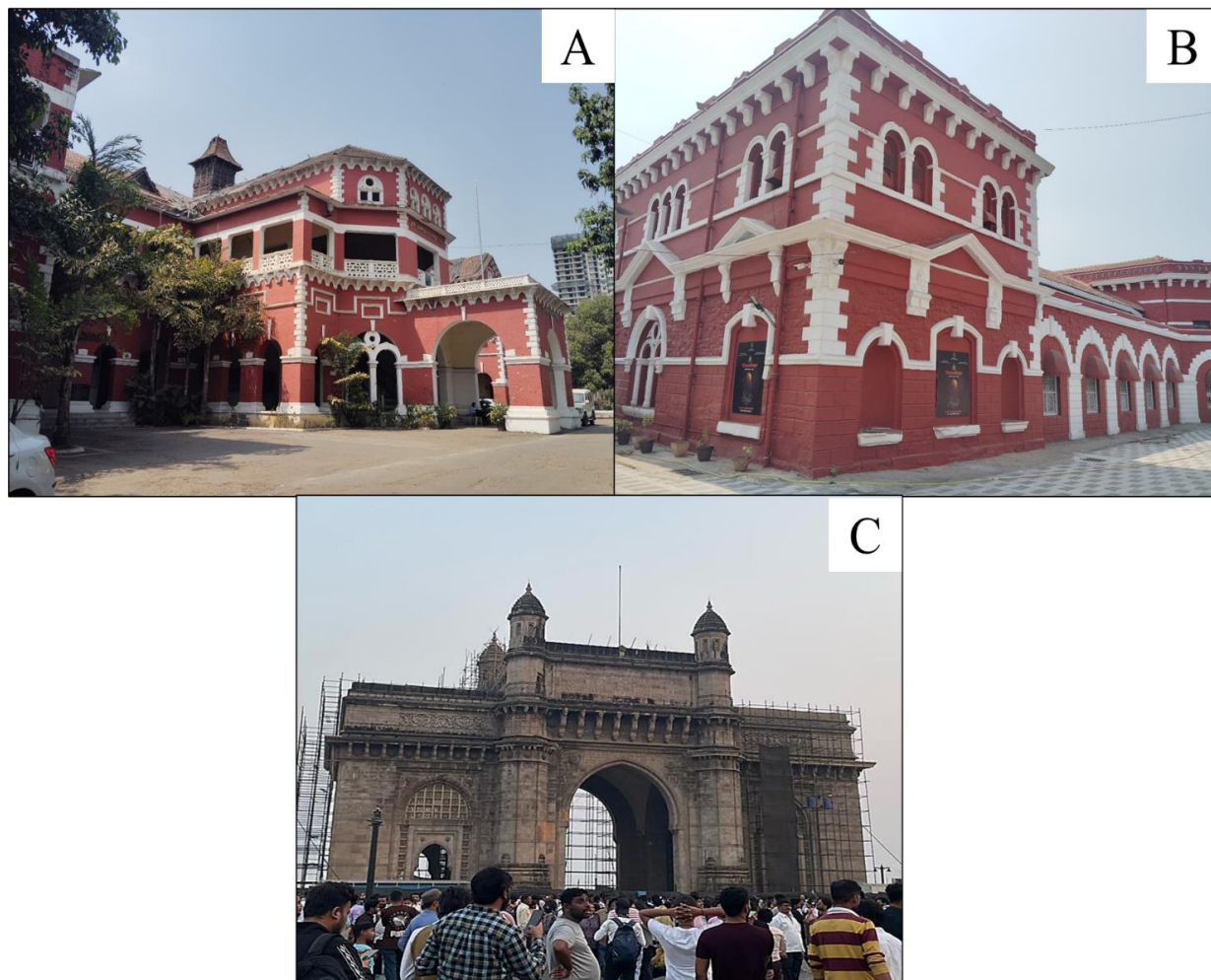
Fig 2: Showing Indo- Saracenic architecture (A): Building of Punjabrao Deshmukh Agricultural university, Nagpur, (B): Nagpur Central Museum, Nagpur, (C): Gateway of India, Mumbai
